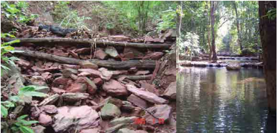
Figure 23: Before (2005, left) and now (right), Samkha reservoir and a check dam network have rejuvenated the community
